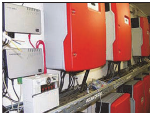
Figure 3 - Radio ripple control, Power Reducer Box and inverters (under installation)
